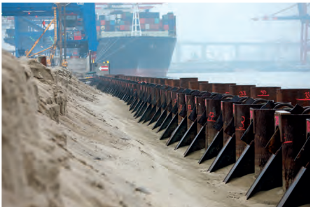
Quay wall construction at Burchardkai
