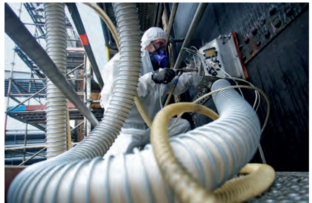
Asbestos clean-up with a vacuum cleaner
